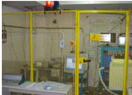
Fig. 1 – The high voltage test room.
