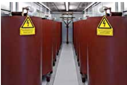
Testing Laboratory for grid integration (Fault Ride Through Container)
