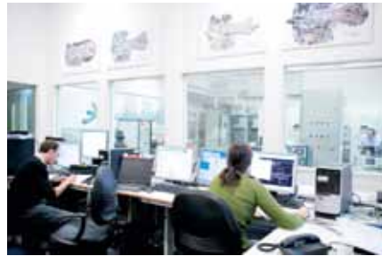
The Intelligent Electrical Power Networks Evaluation Facility (IEPNEF) Control Room
